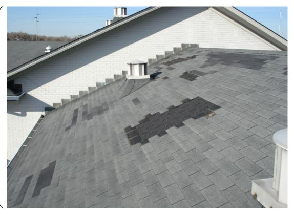
Severe winds passing over this roof caused widespread shingle loss, often in patches, because the shingles were well sealed – holding them together as they peeled and tore from the roof during the storm.
