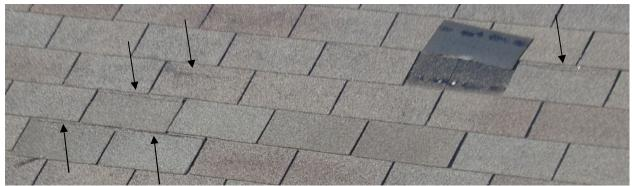
Numerous creased shingles (highlighted with arrows) indicate that they've flapped back and forth repetitively in the wind, probably over a long period of time. Eventually these shingles will tear and blow away, even under mild winds not associated with severe weather.
