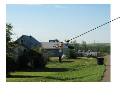
Winds passing over a roof create locally more intense forces of uplift at roof corners, eaves, rakes, hips, and ridges. Severe winds that were parallel to the ridge of this roof induced damage along the rake that extended into the field of the roof.
