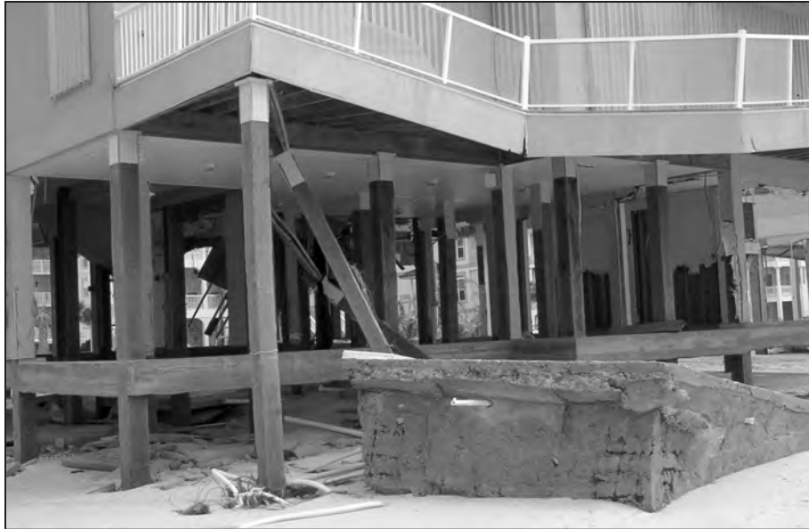
Figure 18. Movement of a spa likely caused failure of two piles supporting an elevated deck.
