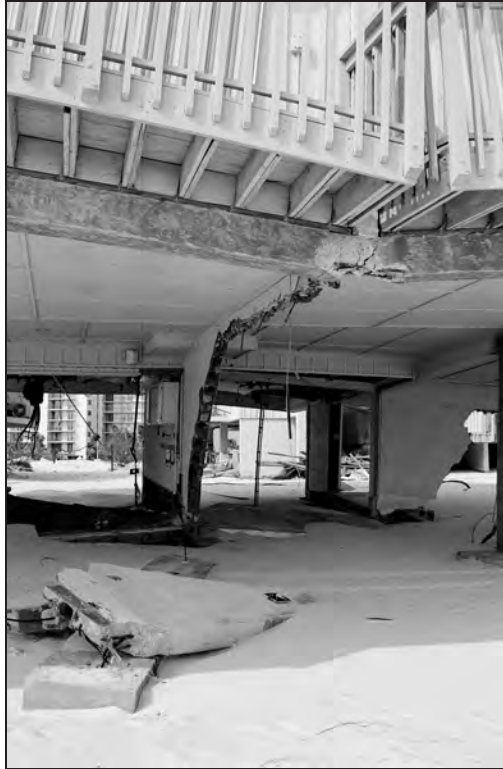
Figure 10. Failure of shore-perpendicular (and shore-parallel) solid foundation walls, and of beam and floor system supported by the shore-perpendicular wall (pre-FIRM structure)
