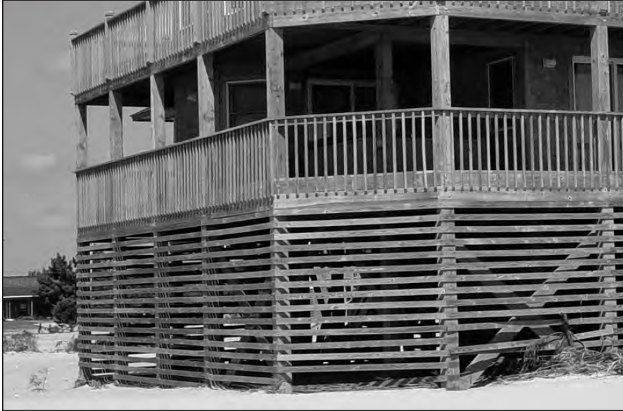
Figure 4. Wood slats installed flat against foundation pilings
