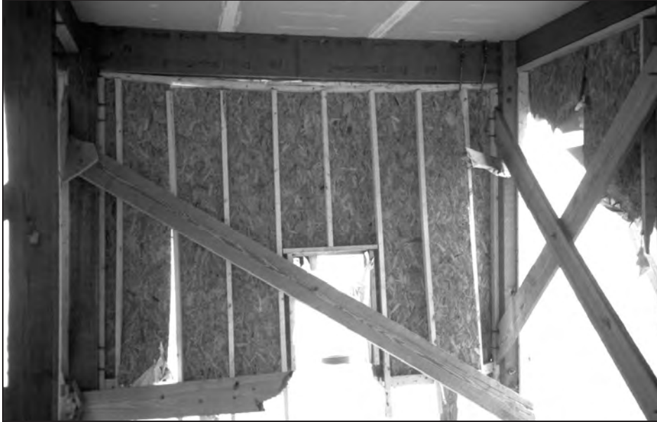
Figure 7. Non-compliant bracing arrangement
