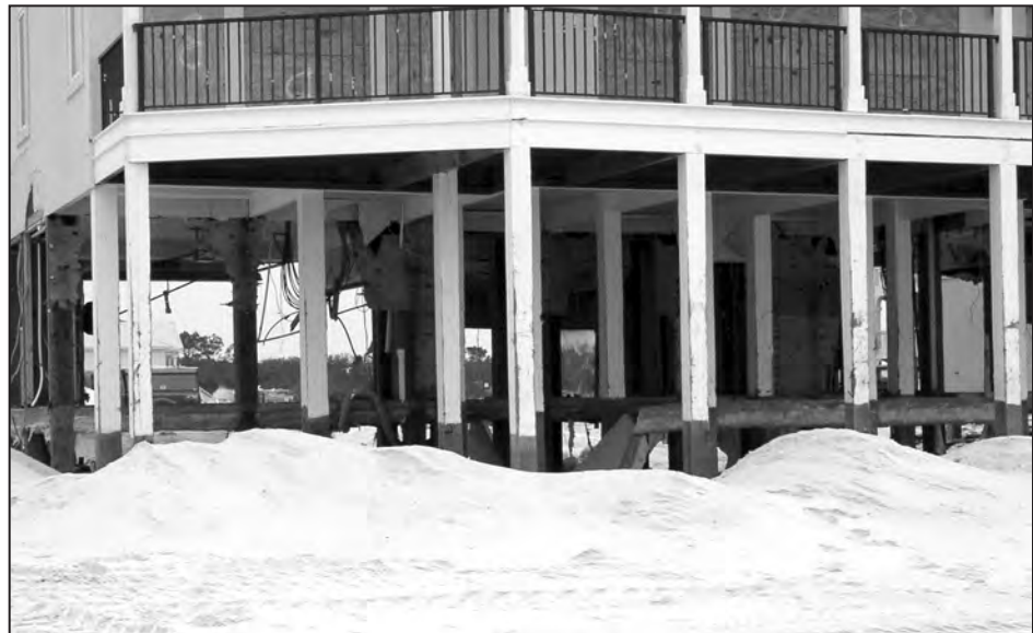
Figure 3. Successful breakaway wall performance
