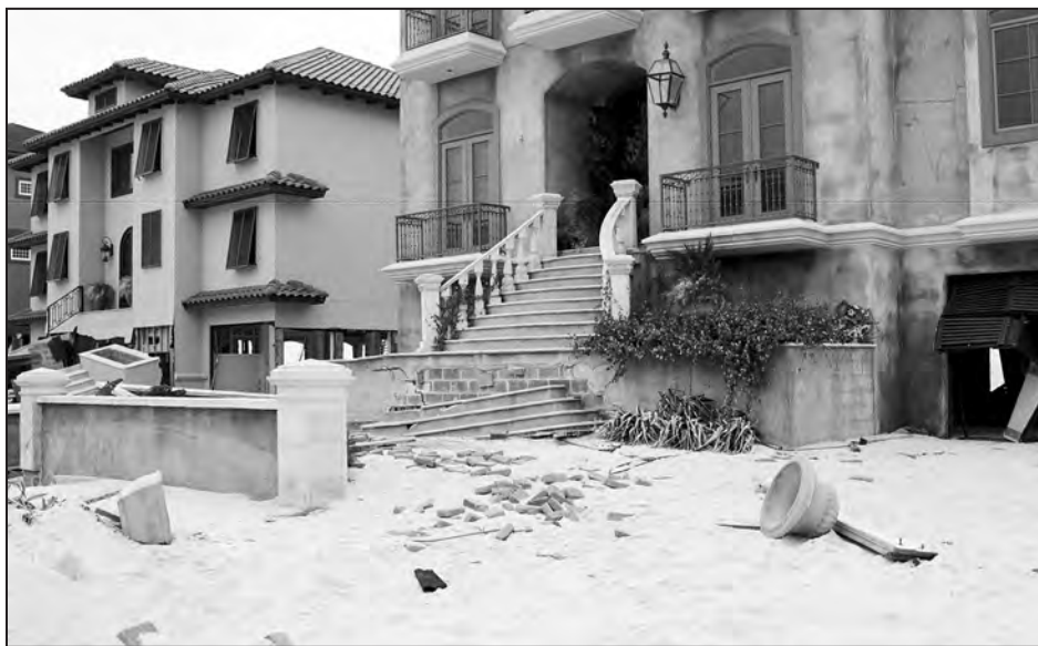
Figure 4. Non-compliant stairs
