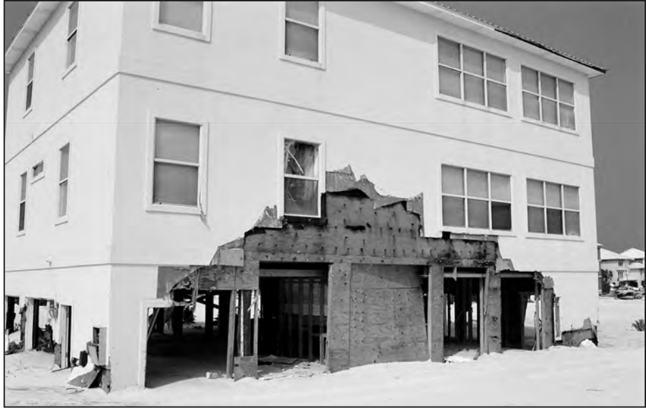
Figure 5. Non-compliant breakaway wall joint detailing
