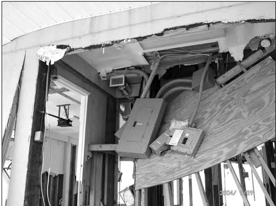
Figure 6. Non-compliant utilities attached to breakaway wall
