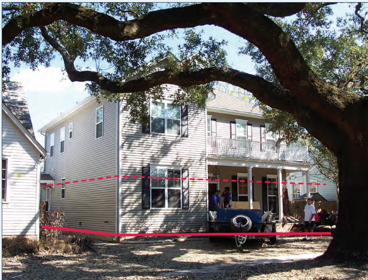
Figure 2-6. Note the actual flood depth from Hurricane Katrina (dashed line) vs. the BFE (solid line).
