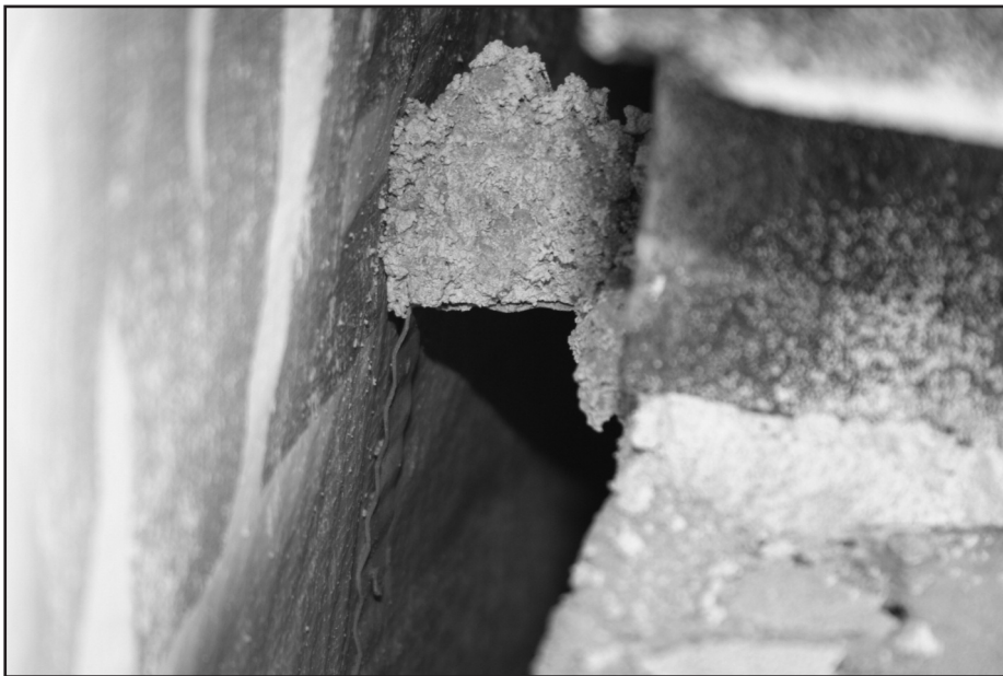
Photo 1 – Mortar droppings collect on top of metal brick ties and bridge the 1-inch air space, coming into direct contact with a highly permeable weather-resistant membrane.
