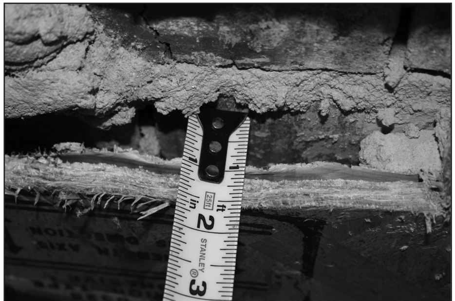
Photo 2 – A typical 1-inch air space ends up being reduced due to the presence of mortar and variations in wall framing and brick alignment.
