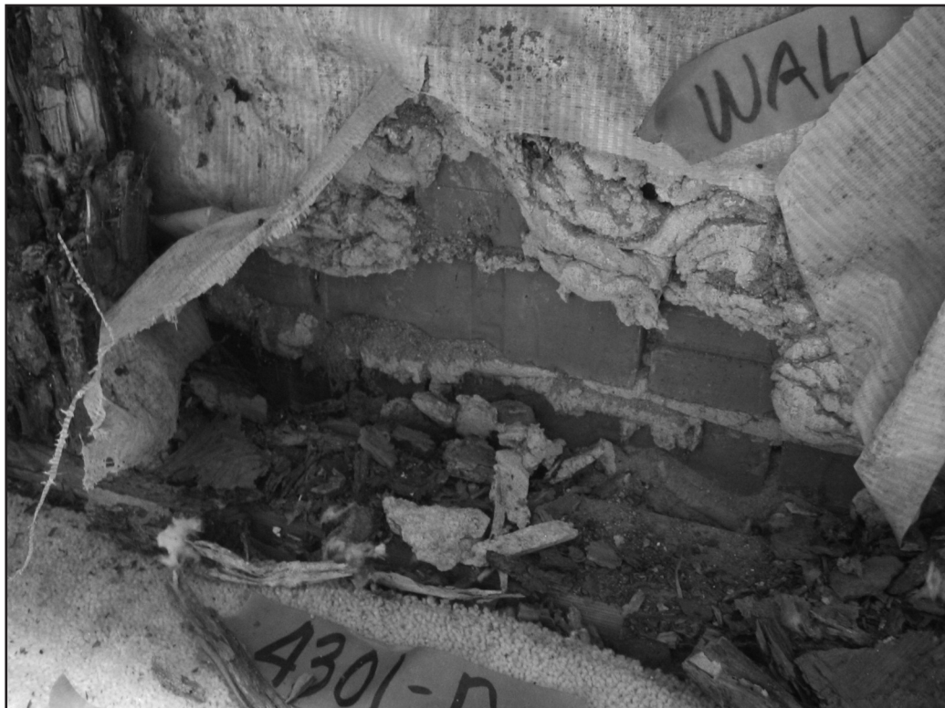
Photo 4 - View of the interior side of the wall shown in Photo 3 that was exposed during destructive testing. Both the exterior wall sheathing and dimensional wood framing members were rotten. An interior-side vapor barrier was placed behind the interior drywall.
