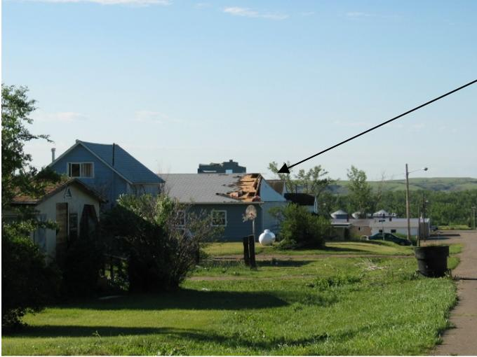
Winds passing over a roof create locally more intense forces of uplift at roof corners, eaves, rakes, hips, and ridges. Severe winds that were parallel to the ridge of this roof induced damage along the rake that extended into the field of the roof.
