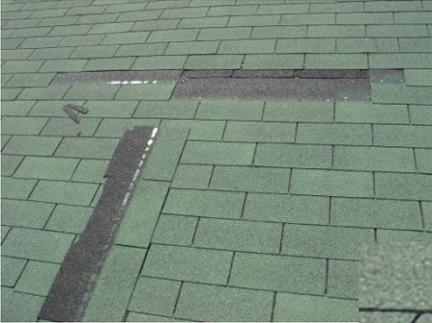
In these areas, the smooth and slick texture and reflective appearance indicates that the sealant strip failed to adhere as designed.
