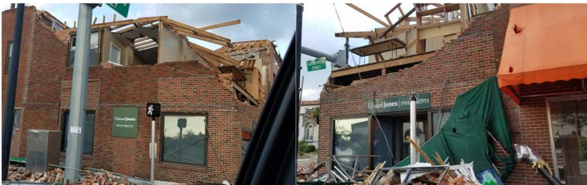
Figure 41: Commercial building (Edward Jones investments) with wall collapsed and roof structure damaged on Lafayette St. in Marianna.
