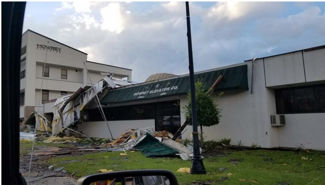
Figure 43. Commercial building (Mowery Elevators) sustaining severe roof damage on Lafayette St. in Marianna.
