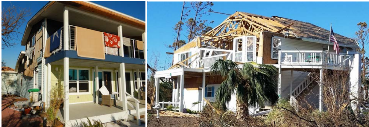
Figure 32: Examples of moderate (left) and severe (right) damage to homes assessed near the intersection of Highways 98 and 386 in Mexico Beach.
