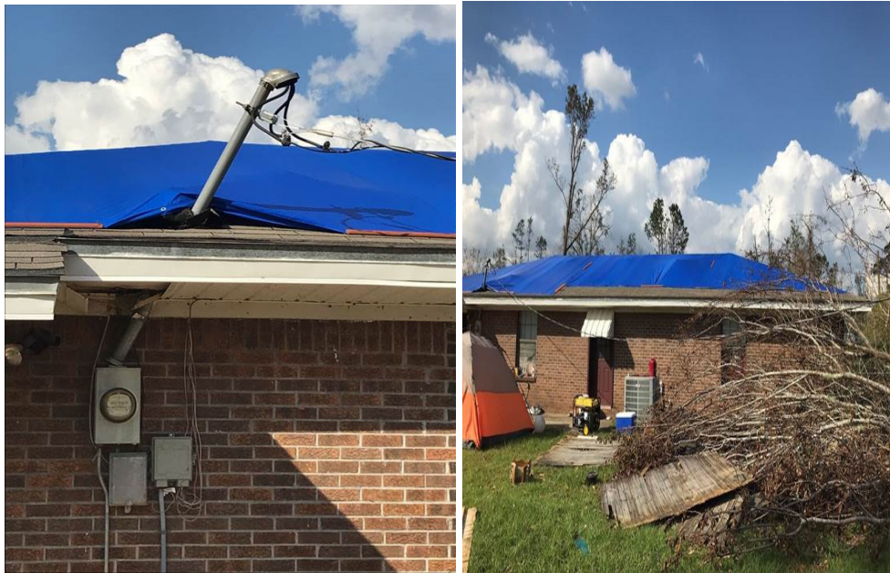
Figure 39: Damaged electricity conductor present in a building near Lambert Ave. in Blountstown.
