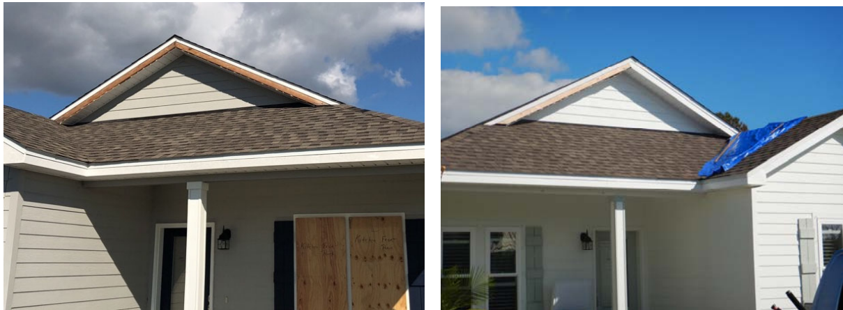
Figure 33: Typical fascia damage of homes in the Beacon by the Sea Community.
