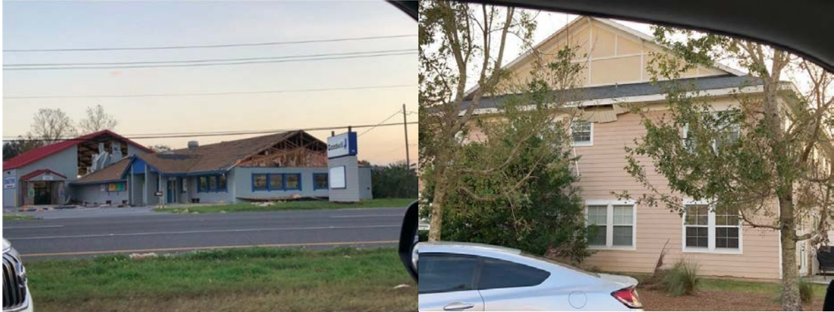
Figure 12: (left) Commercial building in Panama City Beach sustaining severe wind damage. (Right) Multifamily building under construction sustaining minor wind damage in Panama City Beach.
