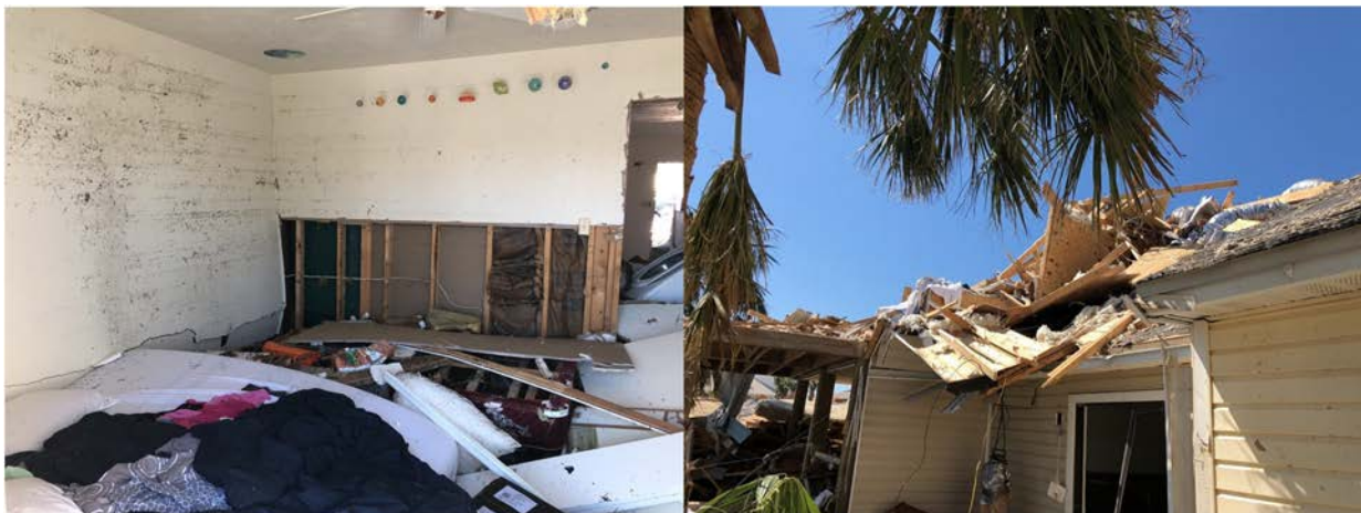
Figure 25: Example of storm surge damage in Mexico Beach. High water mark, 8" short of the 8 ft ceiling, slab is elevated 5" above ground level so surge height estimated 93" AGL.
