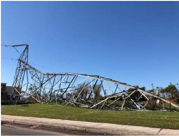
Figure 49: Destroyed transmission tower near North Tyndall Parkway, Springfield (Latitude: 30.160519, Longitude: -85.591164).
