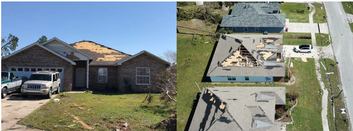
Figure 22: Damage to roof cover and roof sheathing in residential homes in Cedar's Crossing.
