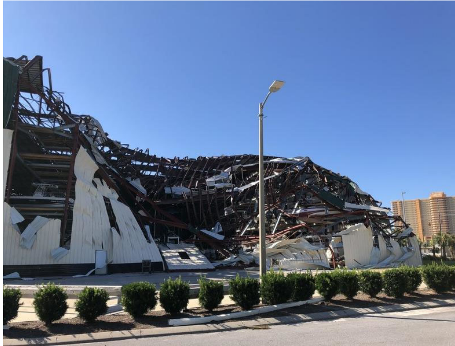
Figure 15: Partial collapse of a metal building marina in Panama City Beach.
