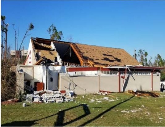
Figure 19: Severely damaged roof at Family of God Baptist Church at 901 US-98 BUS, Panama City (Captured by: Tim Johnson)
