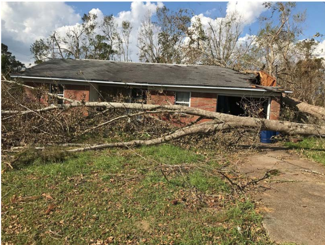
Figure 40: Residential building sustaining severe damage due to tree fall at NE Lambert St. in Blountstown.
