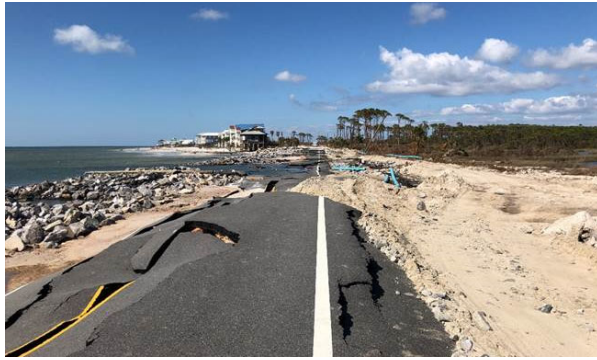
Figure 45: Road washout on Highway 30E (Cape San Blas Rd) on Saint Joseph Barrier Island (Latitude: 29.680619, Longitude: -85.366115).
