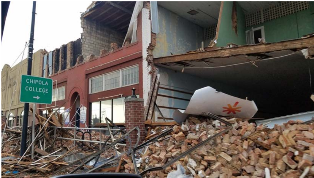
Figure 42: Commercial buildings with masonry walls collapsed and roof structure damage on Lafayette St. in Marianna.
