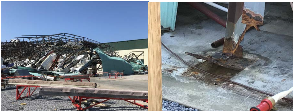
Figure 14: Collapse of a storage building (left) with corrosion and material loss in columns and baseplates (right).
