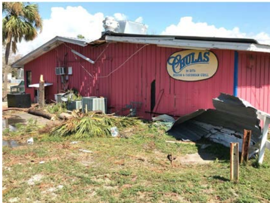
Figure 16: Commercial structure in Interior Panama City Sustaining minor wind damage.
