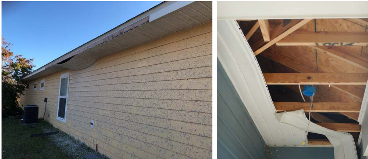
Figure 34: Typical soffit damage to homes in the Beacon by the Sea community.
