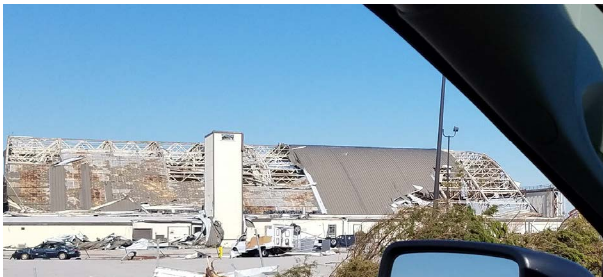
Figure 24: Severe wind damage observed to a large aircraft hangar on the Tyndall Air Force base, with almost complete failure of the corrugated metal roof cladding system.
