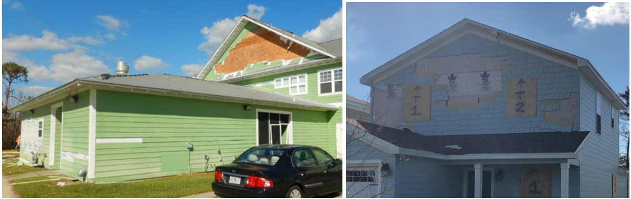
Figure 35: Examples of siding loss in an assisted living facility (left) and single family residence (right) in the Beacon by the Sea community.
