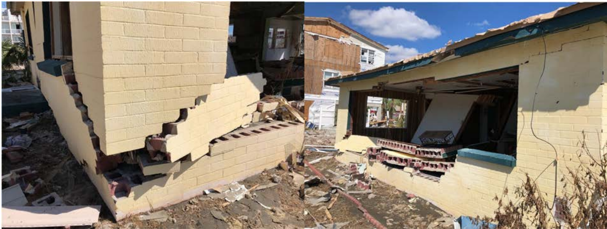
Figure 26: Severe damage to a masonry building observed in Mexico Beach (likely due to storm surge).
