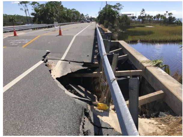
Figure 48: Bridge approach washout on Highway 30A Bridge near Saint Joseph Bay (Latitude: 29.754006, Longitude: -85.303750).
