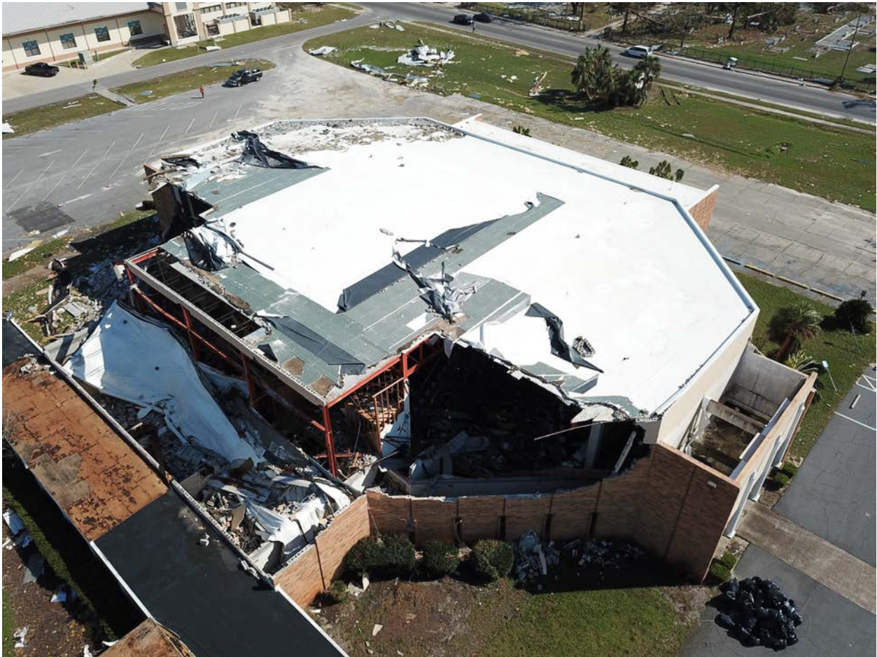
Figure 20: Failure of roof cover and exterior wall of a gymnasium at the Bay County Prep Academy (Lat: 30.16902, Long: -85.67445).
