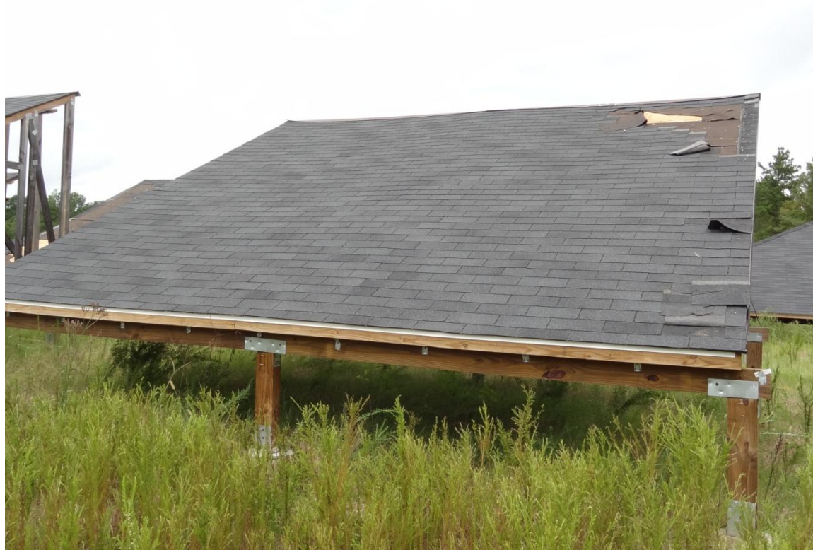
Wind Damage – Science - UF @ IIBHS – Test Facility
