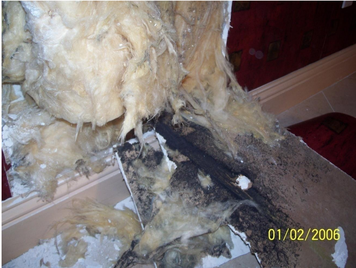
Water Intrusion – Storm Water
