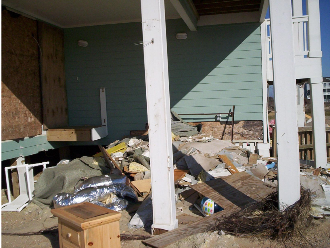
Wind & Flood Damage – Hurricane
