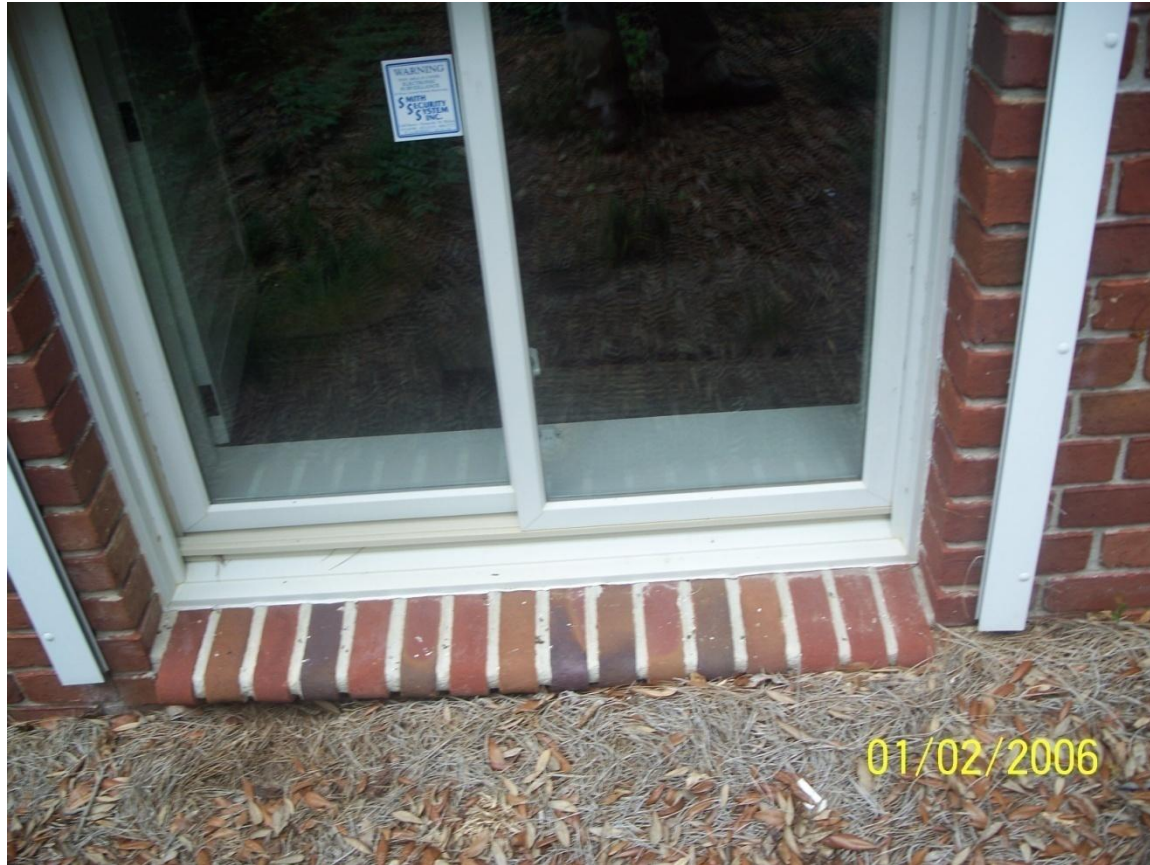
Water Intrusion – Storm Water
