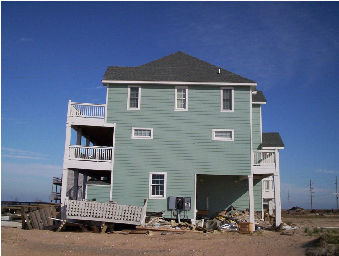
Wind & Flood Damage – Hurricane
